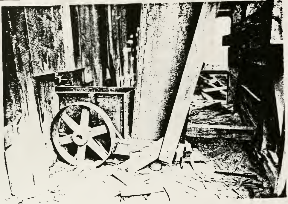
Figure 156. Arsenic plant (structure #56) showing detail of belt lift adjacent to the McDougall roasting furnace, north view.
